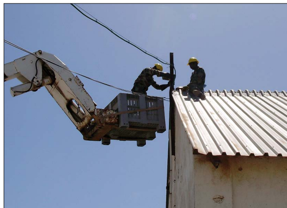
Electrical repair done by Indian Engineers
